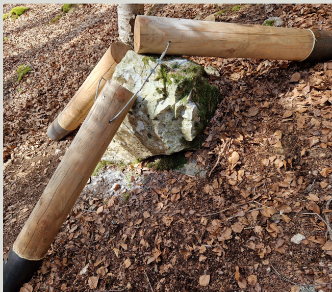
Detail of wooden tripod to fix a loose rock on the surface (OPCC-CTP)
